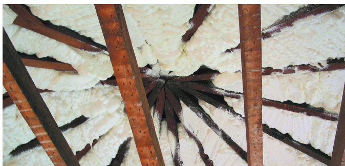
Icynene spray foam can reach and insulate the most complex designs
