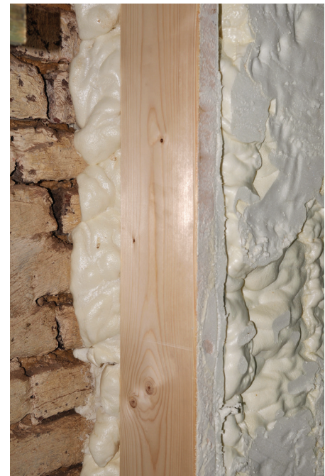
Reduction of thermal bridges
